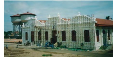
Figure 2 - Chrouy Changwar Water Treatment Plant Expansion Stage I
