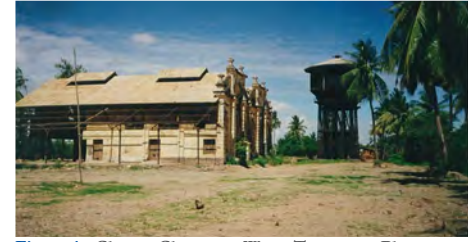
Figure 1 - Chrouy Changwar Water Treatment Plant before 1993
