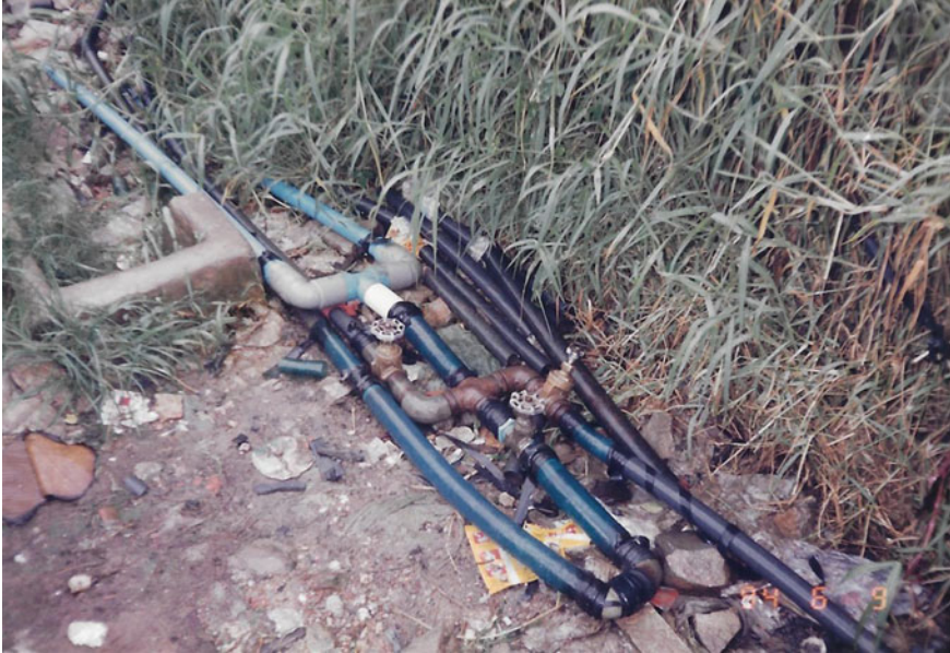
Fig. 3.3 Unauthorised piped connections. Source PPWSA
