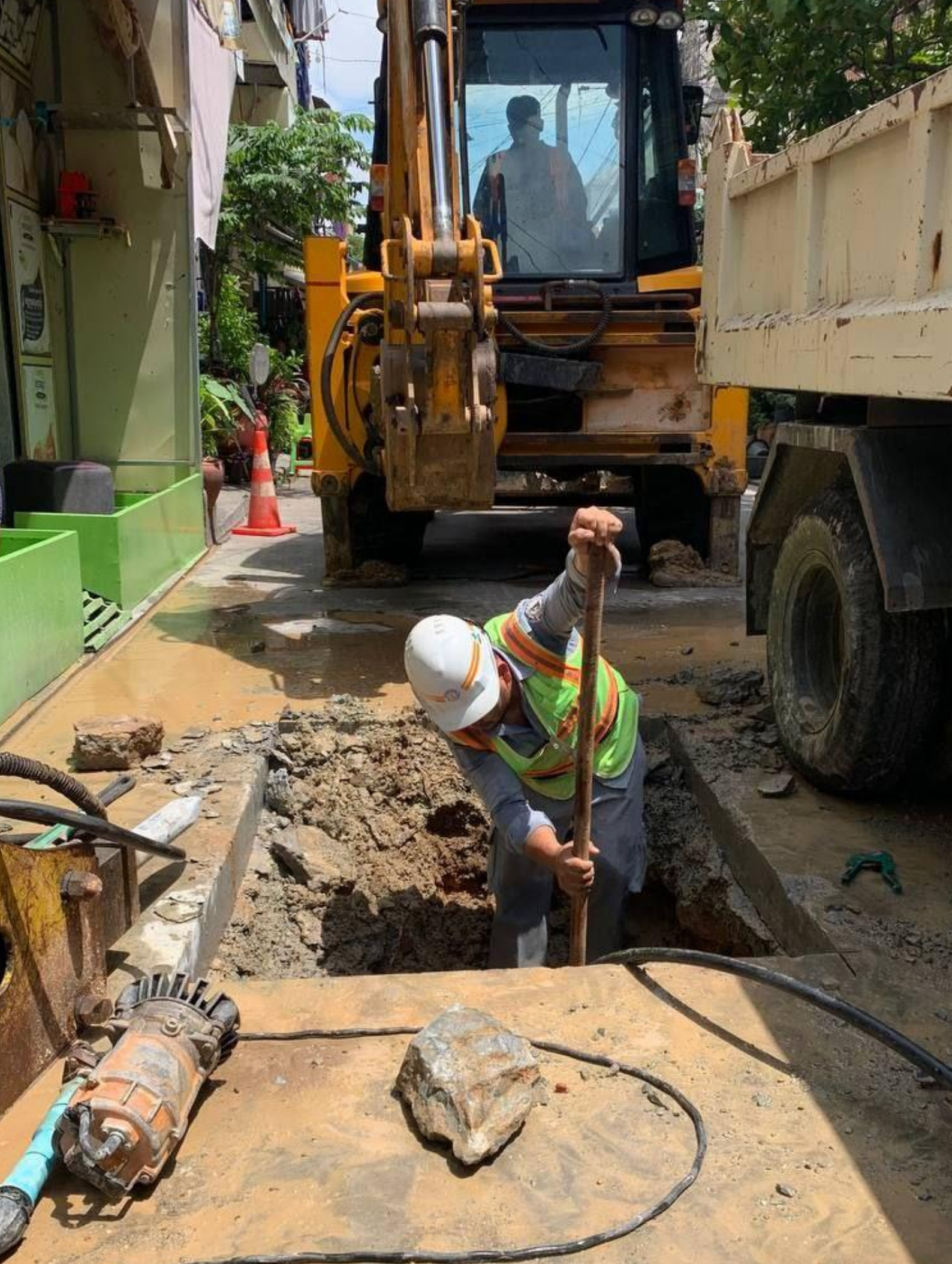
WATER REPAIR AND LEAKAGE DETECTION
